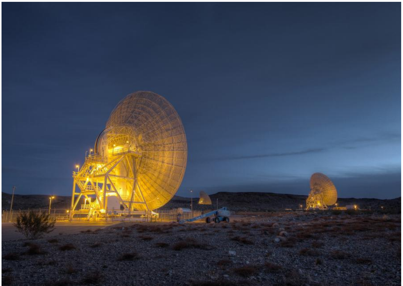
Fig5. Beam Waveguide cluster- an example of how clarity diminishes as distances increase for each antenna until only an indiscernible speck of light.
